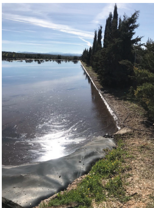
Figure 7.3.4.5: This picture shows the filling level of the third basin and the overflow of the third basin.
